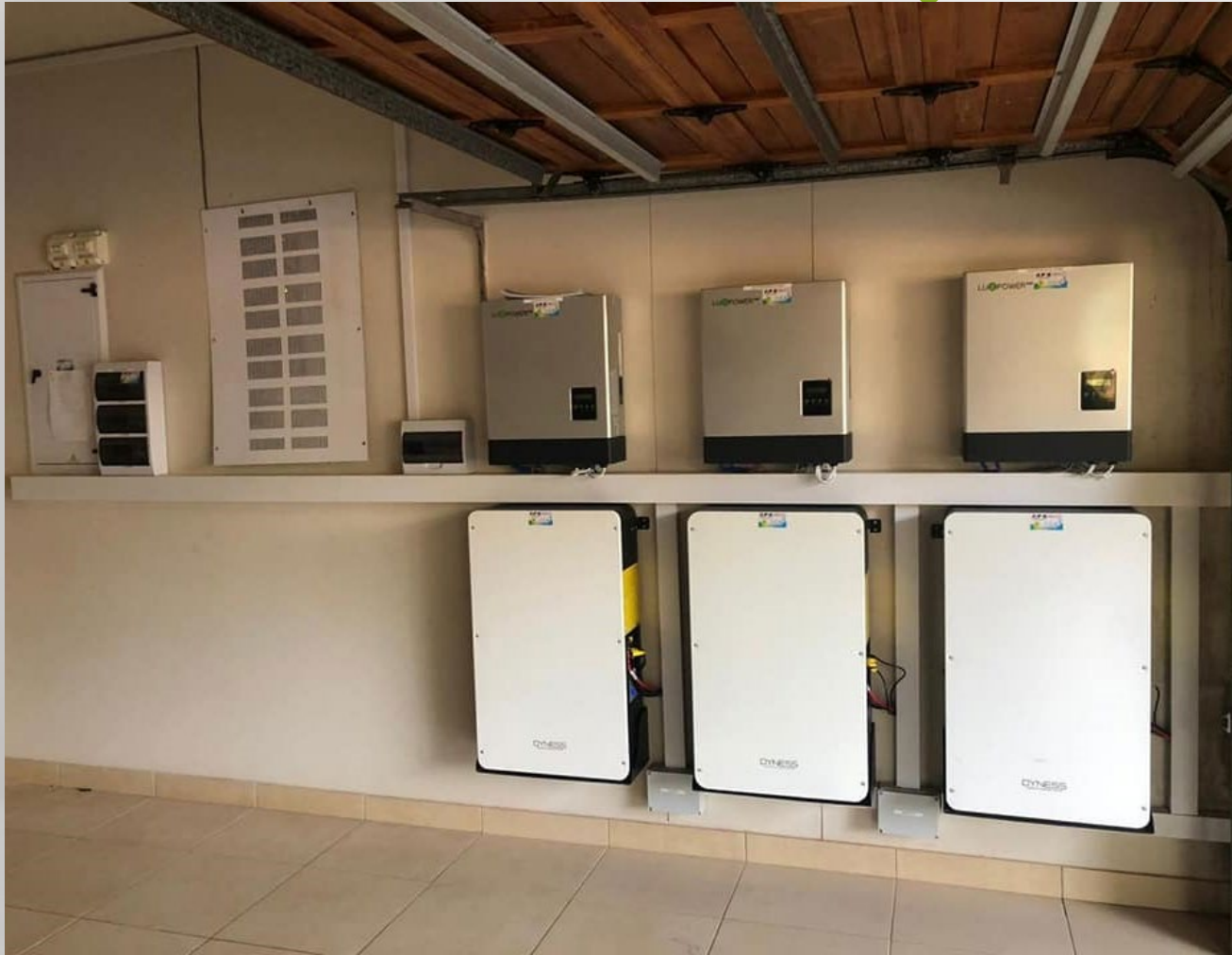
Address: Philippines Capacity: 15kW/28.8kWh Function: Integrated renewable energy
