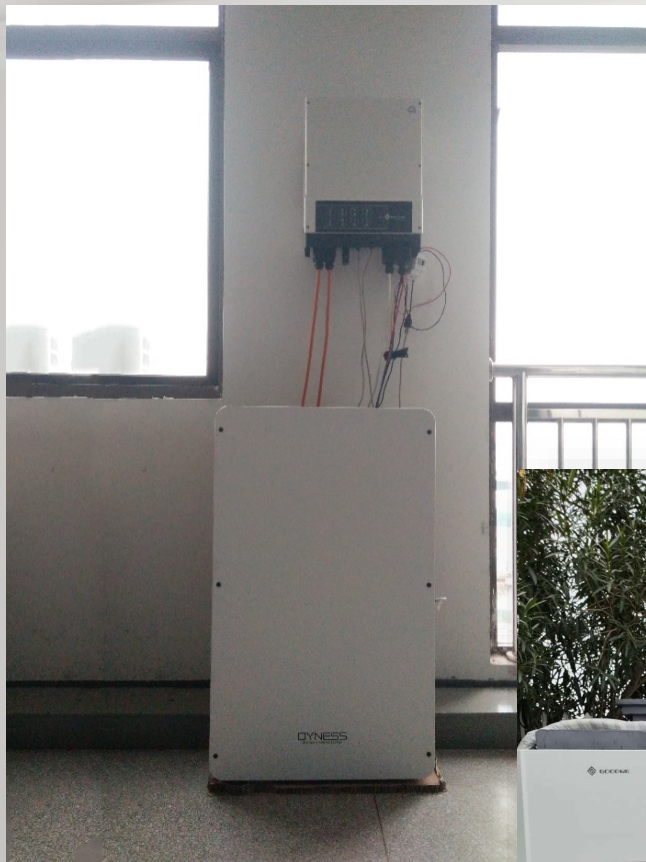
Address: Nanjing Capacity: 5kW/9.6kWh Function: Integrated renewable energy
